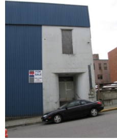
Fig.7 Main Street entrance
