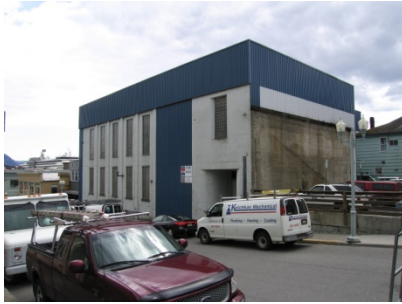
Fig.5 Street view from Northeast
