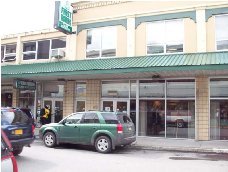
Fig.17: First Bank, Dock Street Data Center on the second floor.
